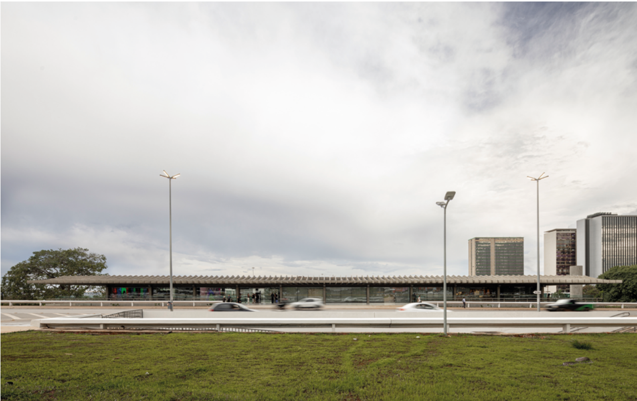
View of Sesi Lab building from L Axis
