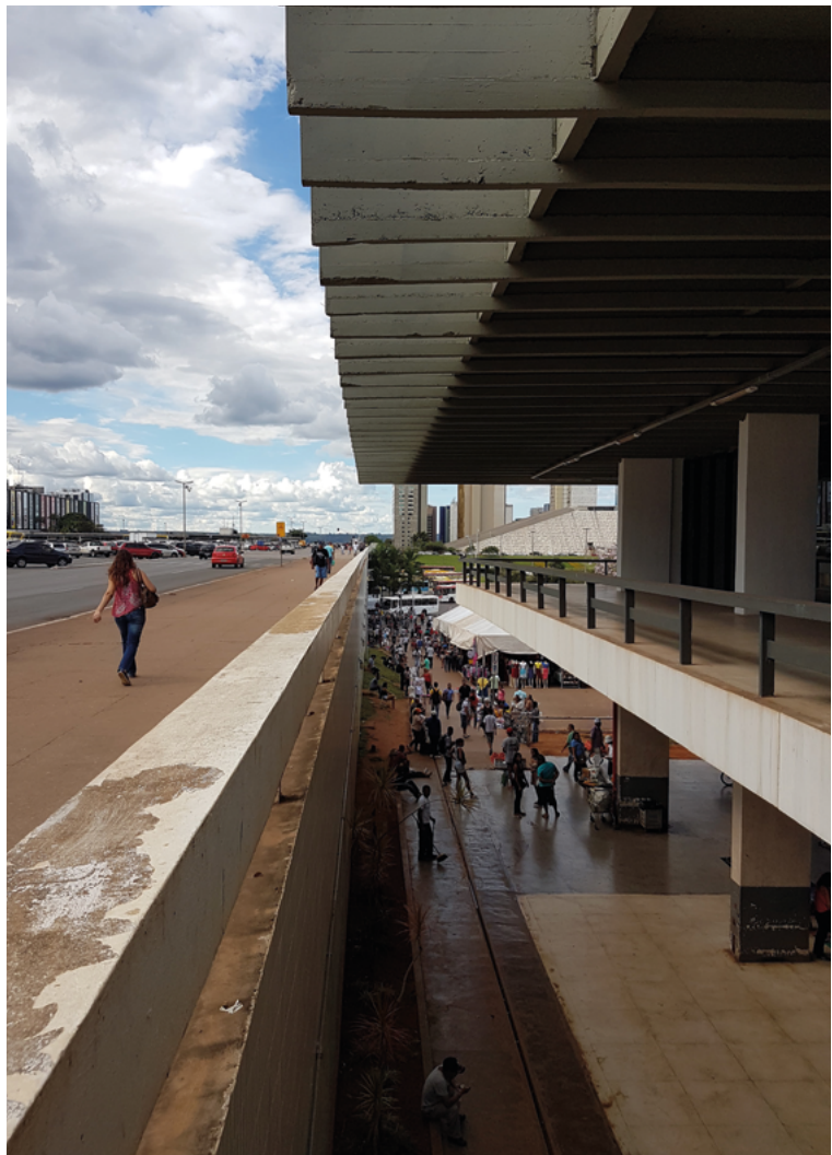
The building being used as an annex to the Bus Terminal. Photo: Cecília Sá
