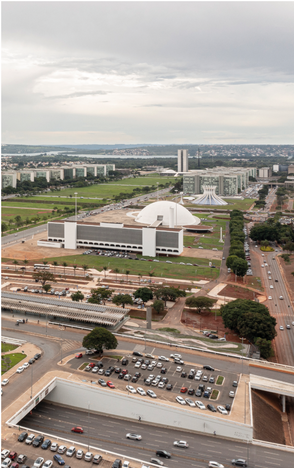
Aerial view of Sesi Lab's building at the junction between Monumental Axis and Thoroughfare Axis
