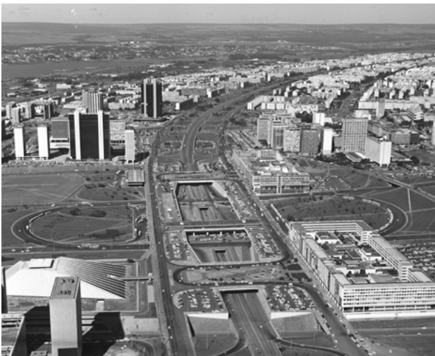
Aerial view of the Bus Terminal Platform with Banking and Theater Sectors, Touring Club do Brasil building (on the left) and Entertainment Sectors and South Commercial Sector (on the right), 1980. Source: Public Archive of Brasília
