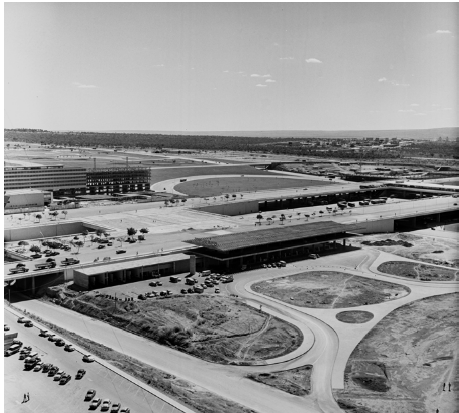
Headquarters for Touring Club do Brasil, Brasília, 1967. Source: Public Archive of Federal District
